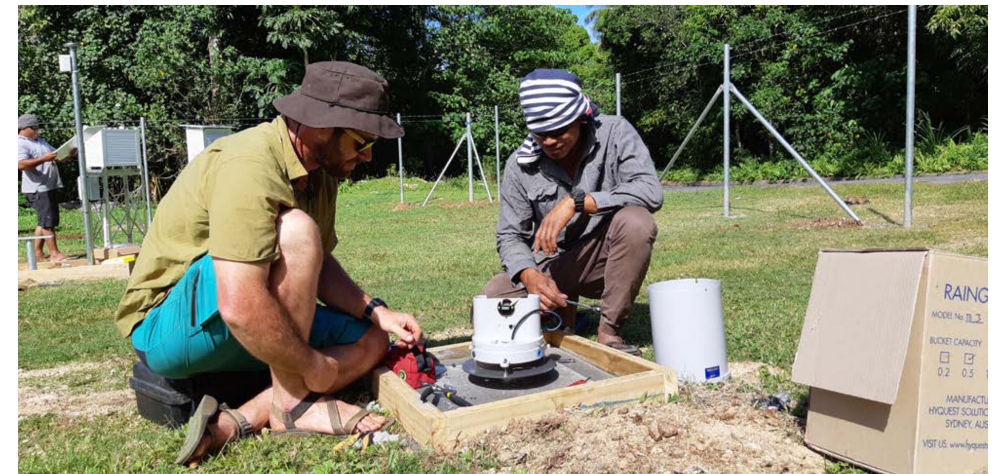
Connecting the sensors. Training is a large part of the Automatic Weather Stations construction and installation process and here Eric Stevens, NIWA Technician, demonstrates the operation of a tipping bucket rain gauge to Tonga Meteorological Service staff. (Jeremy Rutherford, NIWA)
